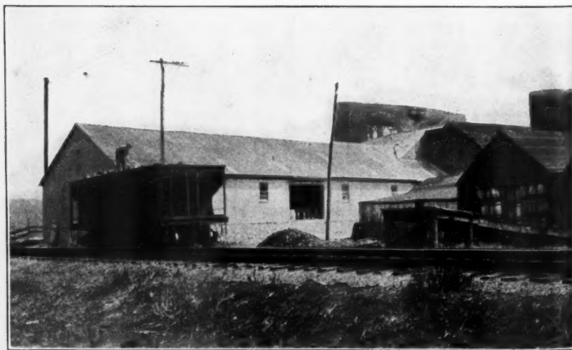
General View of Plant.
